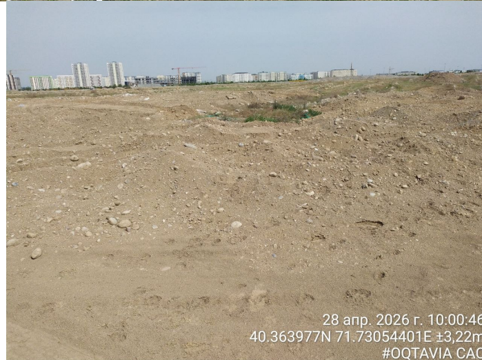
Figure 2: Construction Near the Project Site
