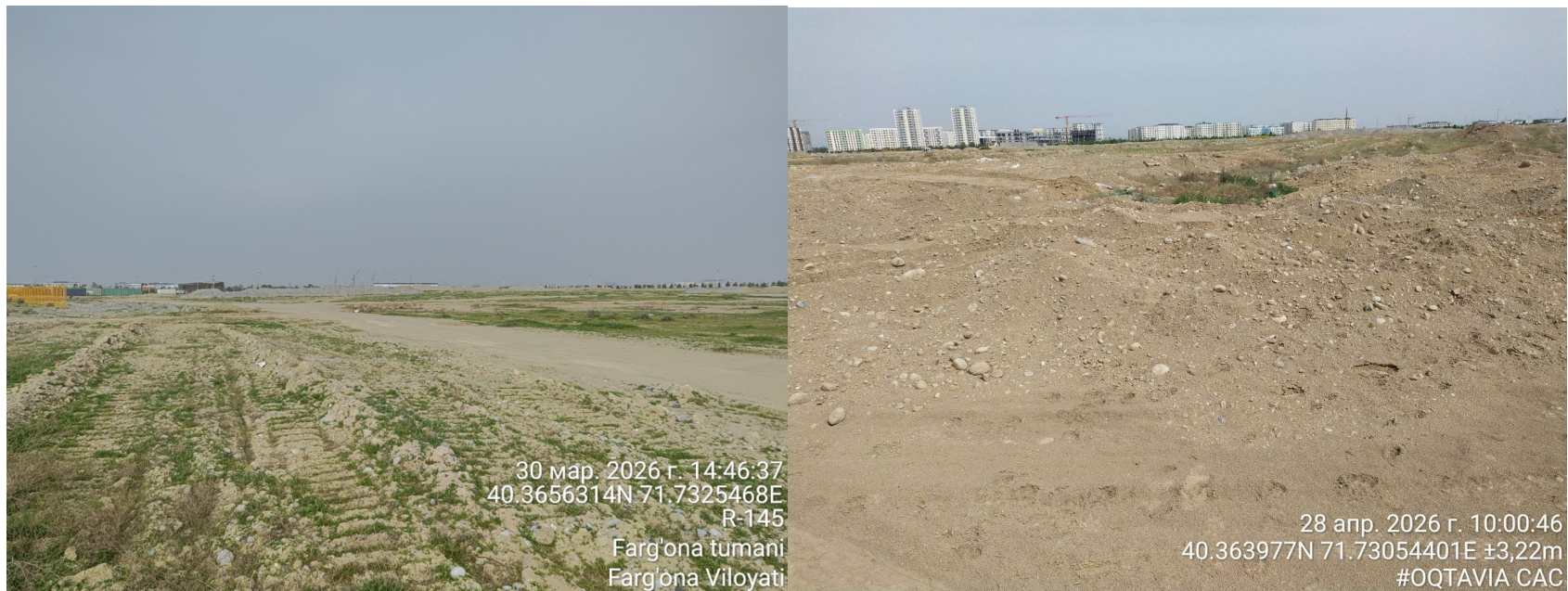
Figure 2: Construction Near the Project Site
