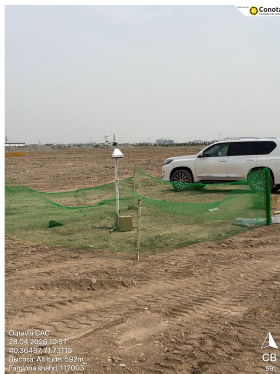
Figure 5: Installation of AQMesh pod
