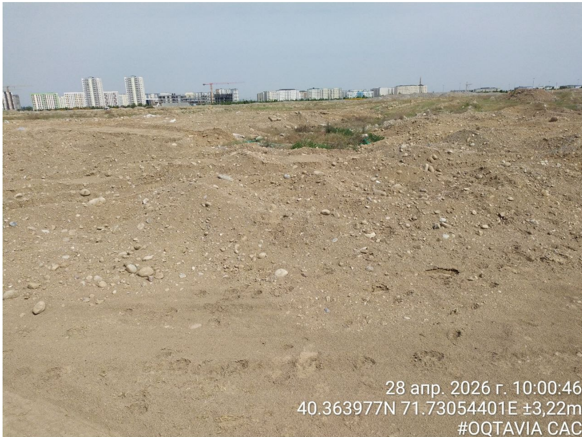
Figure 2: Construction Near the Project Site
